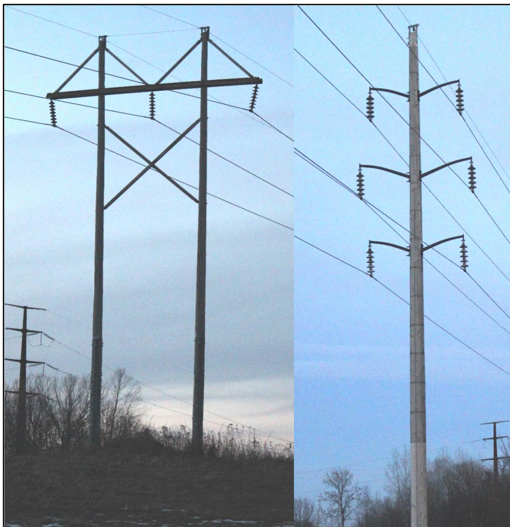
Figure 6-4. Examples of 115-kV H-frame Transmission Structures (left) and Monopoles (right)
