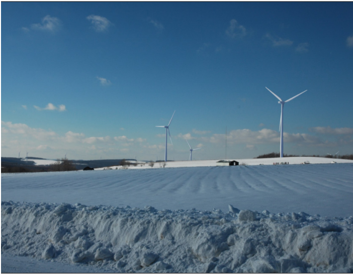
Simulation of "view looking northwest from Kirkwood-Lent Hill Road, Town of Cohocton, NY" (EDR)
