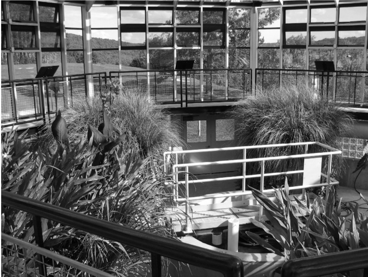
FIGURE 8.11 This artificial ecosystem, known as a Living Machine, treats toilet wastes at a rest stop on the Vermont Turnpike.
