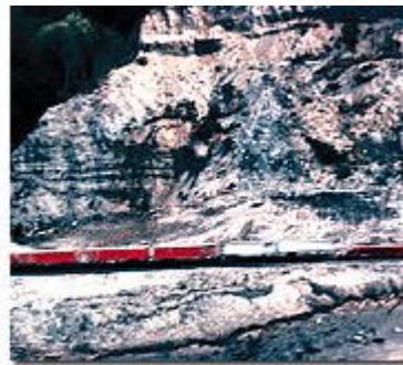
A month later, the track repaired. (Photograph by Ed Harp, USGS.)
