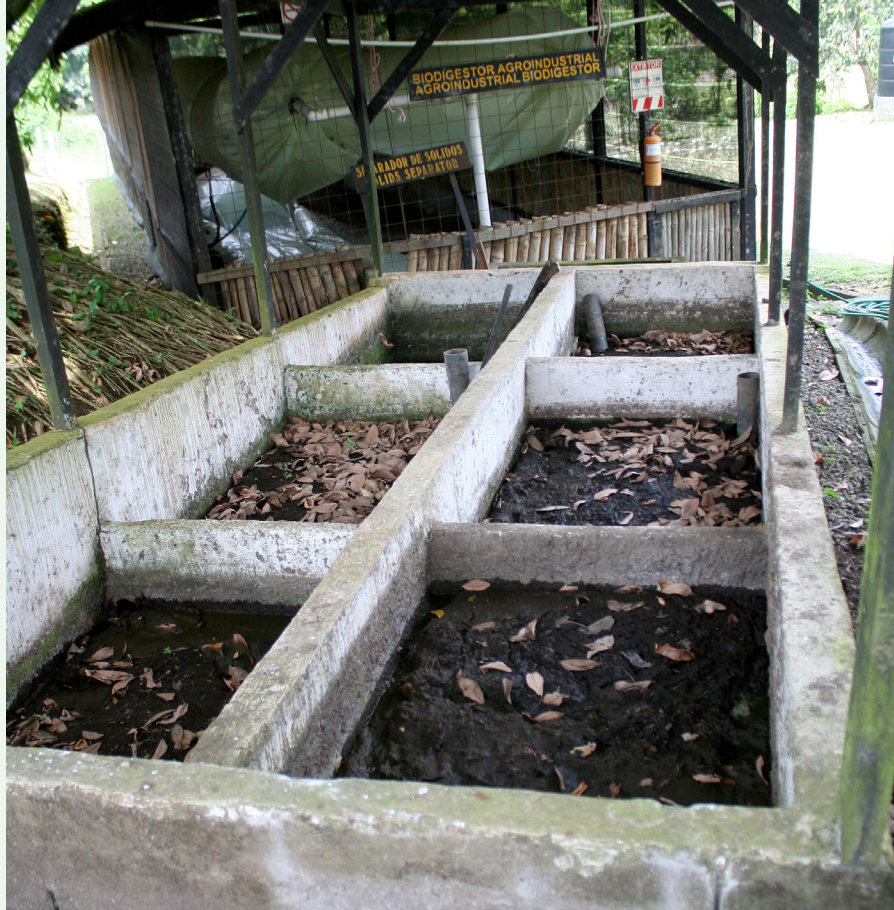
Six biodigesters on the EARTH campus convert animal and human waste to fertilizer and biogas. Over the past few years, EARTH has also installed more than 2,000 biodigesters for farms and businesses around Costa Rica. © 2013 Wendee Nicole
