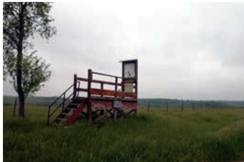
Seven-Mile Creek Viewing Platform.
