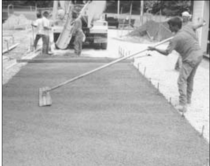
Porous paved driveway at Southface Energy Institute receives its “smooth” coat.
