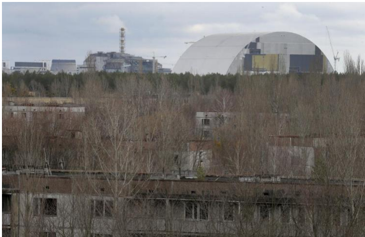
A chimney over the destroyed reactor at the Chernobyl nuclear power plant (background left) and a gigantic steel-arch under construction to cover the remnants of the exploded reactor in the town of Prypyat close to Chernobyl, Ukraine. Houses in the foreground were abandoned by Chernobyl plant workers a few days after the explosion. Since then, Prypyat has become a ghost town. File/Efrem Lukatsky/AP
